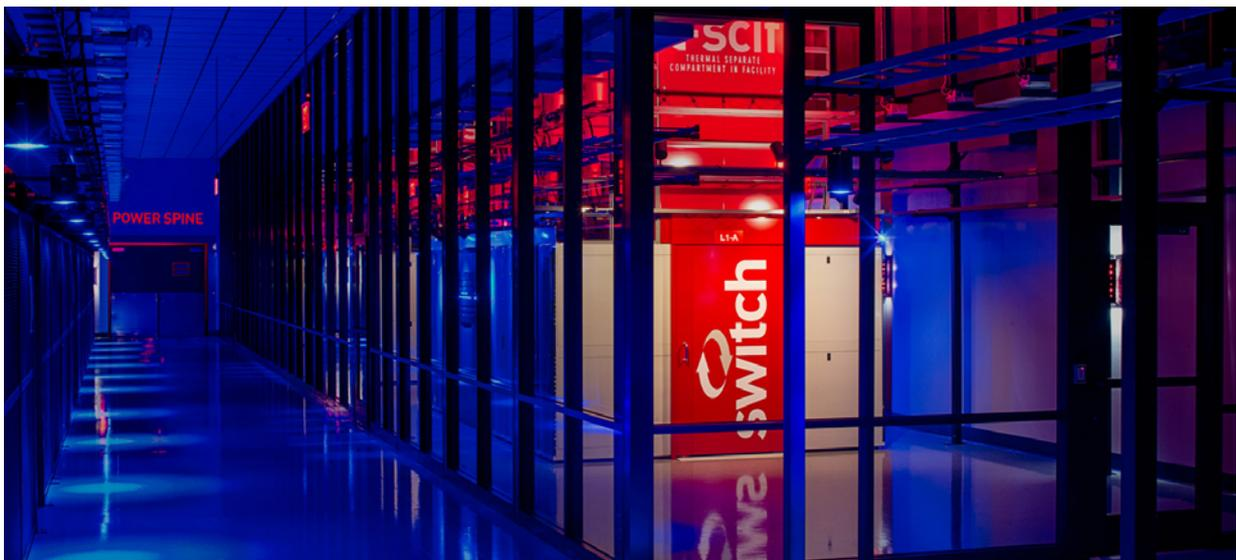
In addition to electricity monitoring, SUPERNAP made material interventions in the cooling service, through the use of T-SCIF (Thermal Separate Compartment in Facility) technology, which maintains 100% separation of the hot air, created by the servers, from the cold air, provided by the TSC500, through a hot aisle and dedicated plenums. TSC500 is the 'smart' HVAC system, also patented by Switch, which makes cooling more efficient.
